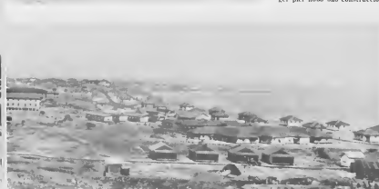
THE ADMINISTRATION Building, No. 1 Powerhouse and expanded community date the above photo to pre-1930 vintage. E EDIFICIO di administracion, No. 1 Powerhouse y cominidad extendi ta muestra cu e retrato aki ta di promer cu 1930.
